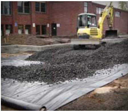
Geotextile provides separation between the soil subgrade and subbase material
