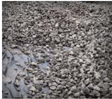
The subbase No. 2 stone provides surface infiltration and vehicular support
