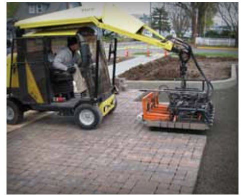
Mechanical paver installation reduces time and cost
